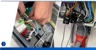
P3 Wallbox Benchmark highlight: As the only wallbox in the test, the zappi enables control of the dynamic charging current and regulates the charging current with the installation of CT coils (measuring units, included in delivery) based on the real-time consumption of P3 Energy.lab. With the retrofitting of the external sensor harvi, the data of the measured consumption can also be transmitted wireless.
